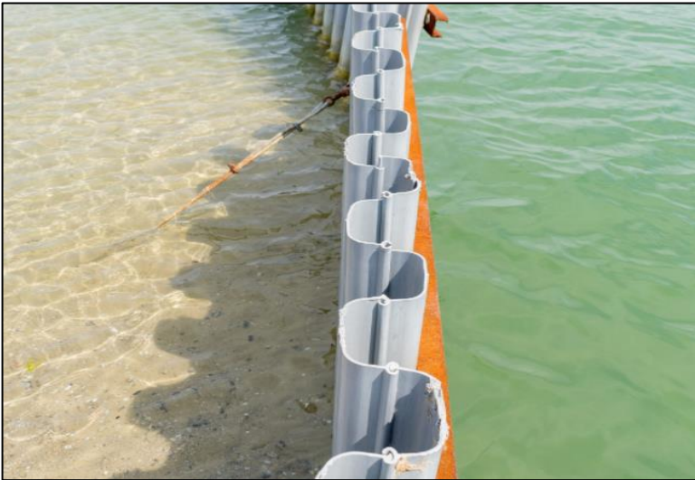
Figure 8: A Typical Cofferdam
