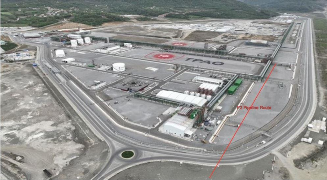
Figure 7-6: Drone image of SGFD SITE Onshore Facilities, Campsites, Sazköy and Planned Phase-2 Pipeline
