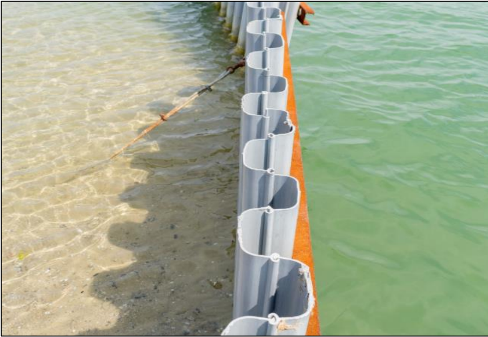
Figure 3-17: A Typical Cofferdam (Source: Phase 1 EIA Report)
